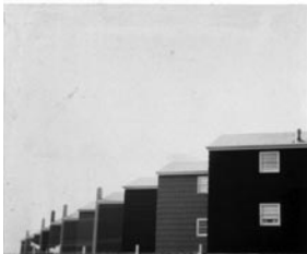
Housing Development, four units, Orange, New Jersey
