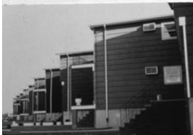
Housing Development, four units, Orange, New Jersey
